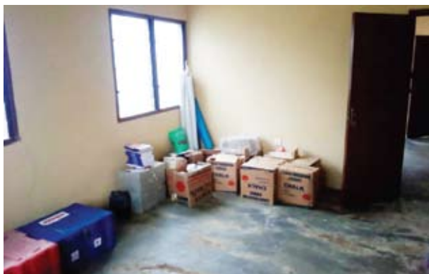
Quality of concrete could not be guaranteed to be as specified since no quality check on concrete was carried out. Valuation for payment was based on the quantum of work, not quality of work especially concrete works.
