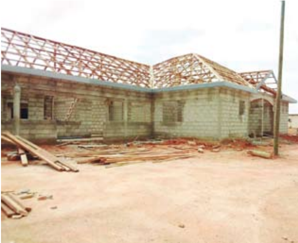
The site ought to be hoarded from the public.
