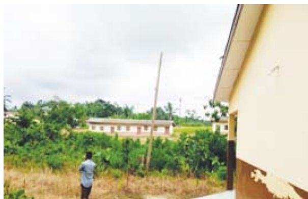
This newly built school block like the existing old school blocks has no provision for urinal and toilet for the pupils.
