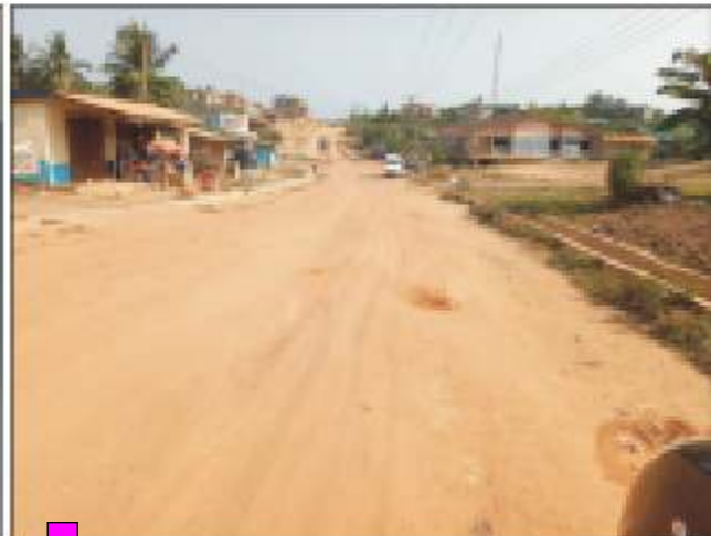
Road need frequent watering to avert the effect of dust from road surface on life and property
