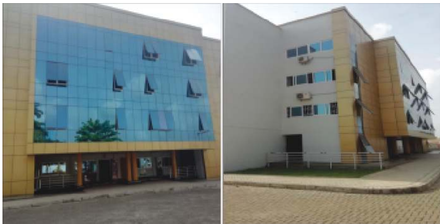
Picture 4: Takoradi library complex
