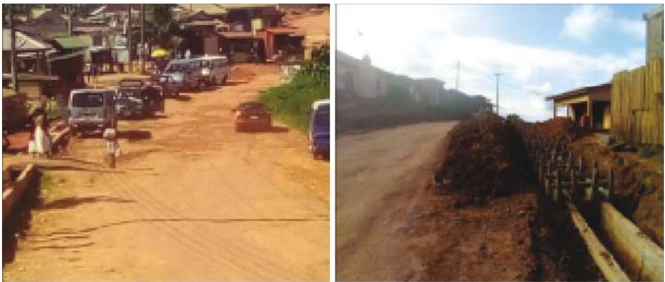
Picture 5: Lot 2 road and drainage works
