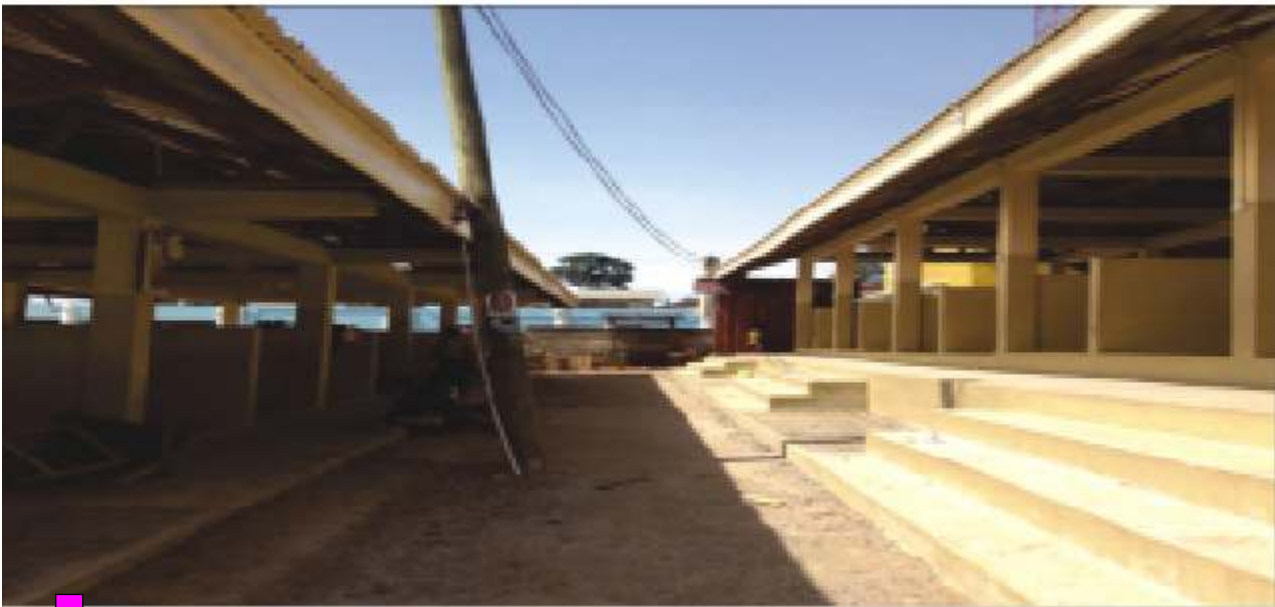
Picture 3: Kojokrom market sheds, now and before
